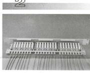
Align the cables with their respective IDC connecting blocks in order of termination. Provide extra cable length for termination-at least 5-10 cm (2-4 inches).
