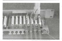
Place the wires into the IDC connecting blocks according to the color code on the blocks. Punch the wires down with an impact tool in order to terminate them. Do not forget to terminate the drain wire if it has been inserted into the ninth slot.
