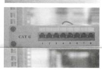
Mount the patch panel in the desired position on a relay rack.
