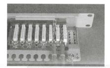
Fasten the cable to the strain relief tabs with cable ties and trim off the excess cable tie.
