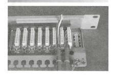
Instead of wrapping the drain wire around the foil shield, the drain wire may be inserted into the ninth slot (the slot with no color code) on the IDC connecting block as shown.
