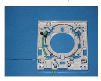
Placing 1st pigtail and splice
