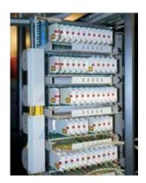
With its modular optical fibre technology, 3M offers the user a complete system for central optical fibre distribution frames with high fibre counts.
